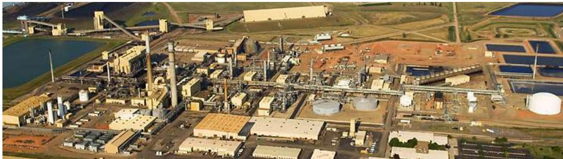
The plant also produces ammonium sulfate, anhydrous ammonia, phenol, cresylic acid, methanol, and naphtha. These materials are by-products of the coal gasification process and are sold as feedstock to specialty chemicals companies. All these by-products are separated and stored in large storage tanks prior to being sold and transported. The products are transferred from storage tanks to trucks or rail cars via load-out systems.
